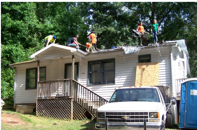
The SOS team repairs and reroofs this house in Henderson.
