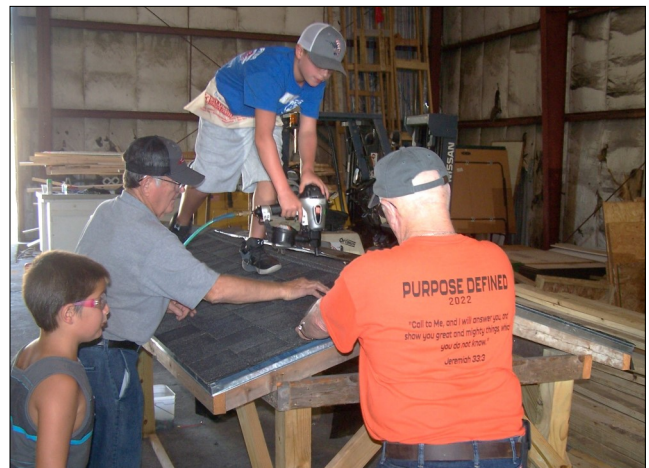
Campers take turns on the "roof" to learn from Cliff McClanahan (left) and Tim Jenks how to nail shingles.
