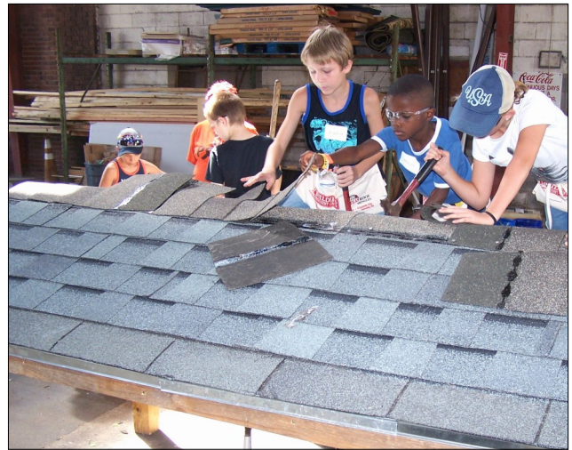
Youths attending Rebuilding Hope's 2023 Kids' Construction Camp work together as they learn to repair a roof.
