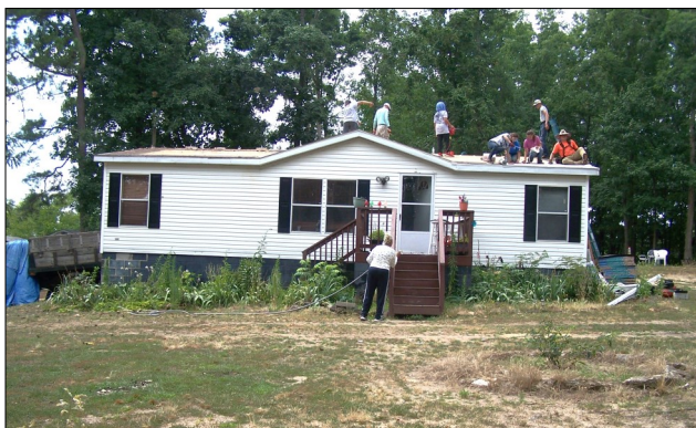
The Ladder Leapers’ job is in the Finch Road area.
