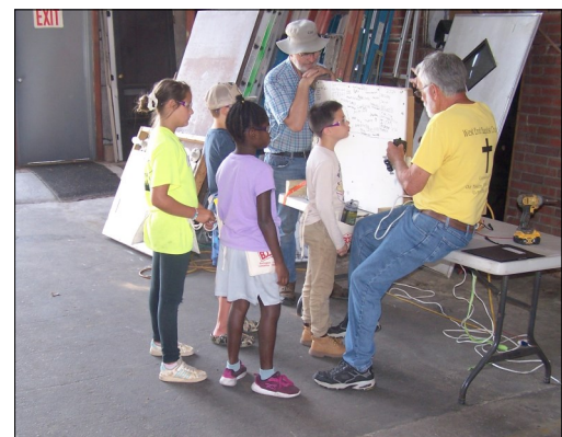
Leon Dillard (right) teaches campers how to make simple electrical and plumbing repairs.
