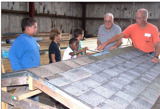
Billy Layton (right) instructs campers in how to remove and replace shingles.
