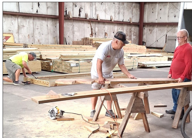
Rebuilding Hope volunteers James Deans, Morris Aycok and James Bean cut and assemble components of a landing and steps for a resident in the Manson area.
